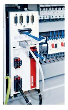
The AX5206 2-channel Servo Drive also contributes to the compact machine design.
